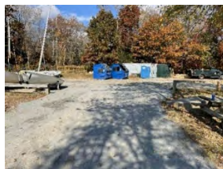
West Lot Flooding Repair 2024
