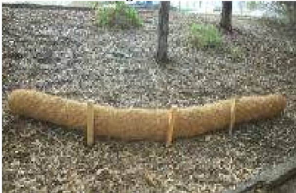
Coir log after Installation
