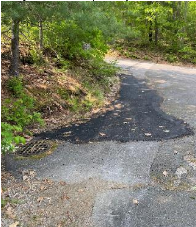
Existing trench drain and repairs to infiltration basin
