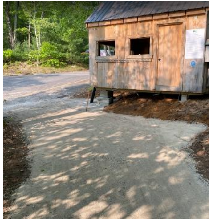
Corrective actions for Sherborn Yacht Club erosion control during boat-house project in 2023
