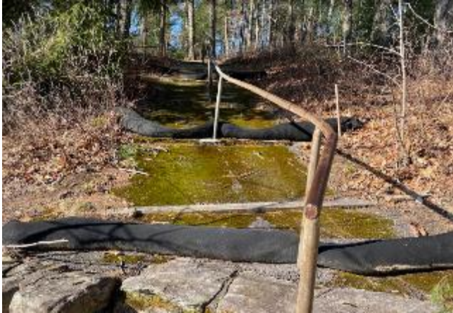
Temporary erosion control in place on the Town stairs from the parking lot in 2024.
