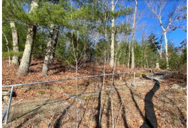
Town-installed pervious stairs to reduce runoff, with additional erosion control and water routing coir logs.
