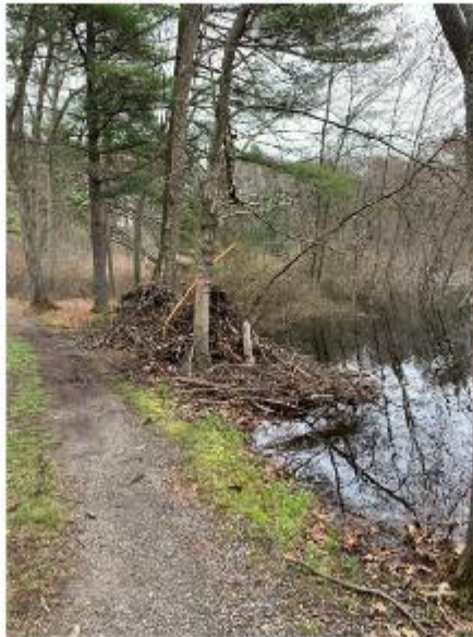
View to east, along cart path. Beaver debris close to culvert. Lagoon along right of path.
