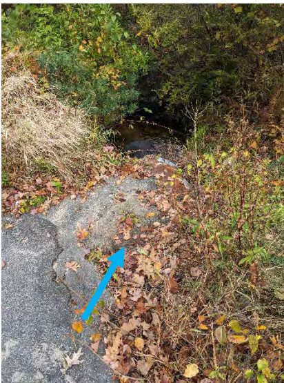
Photo 9-1: Erosion at the culvert outlet at Carpenter Road.
