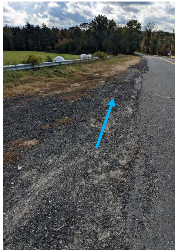
Photo 14-2: Loose sediment along the eastern shoulder of Upper Palmer Road.
