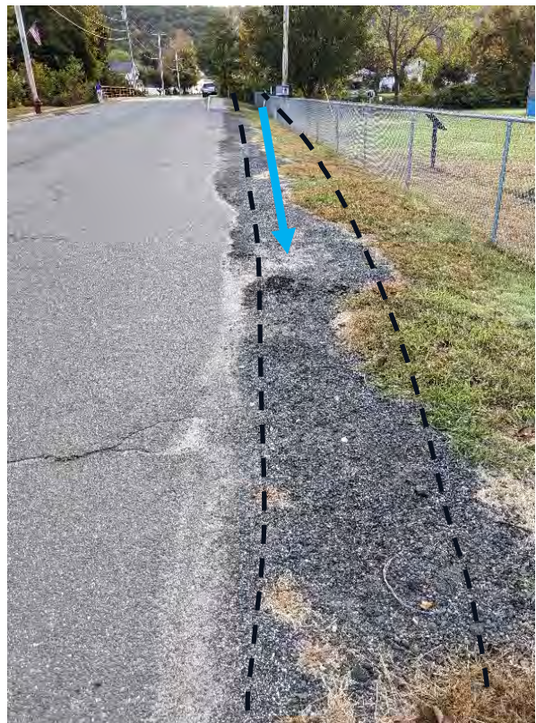
Photo 3-2: Runoff from State Street flows through the gravel shoulder and onto Veterans Field.
