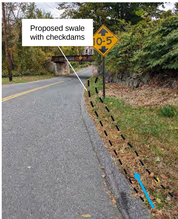
Photo 6-2: West side of Bliss Street.
